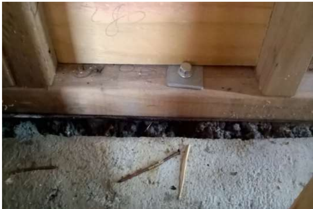
Poorly set out foundations resulting in the building being too small; site concrete added to edge of floor slab. Among other things this will lead to moisture ingress.
