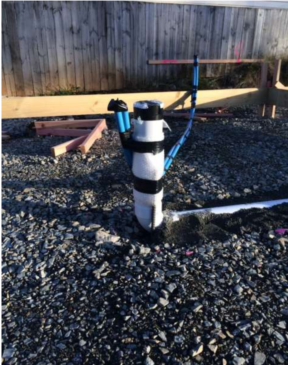
Lack of protection to waste pipe
