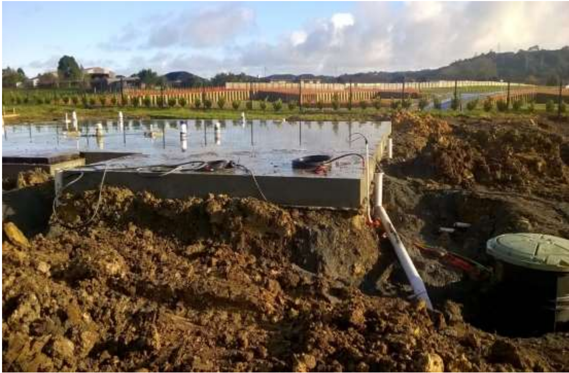
Drainlayer's often undermine the foundations of the building by excavating too close to the building
