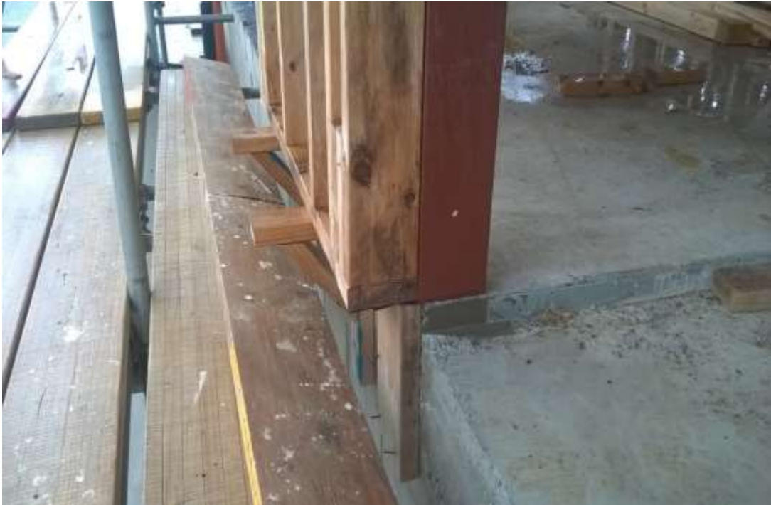
Poorly set out foundations leaving inadequate room to attach the bottom plate, which should be sitting on the edge of the slab not overhanging it as in the photo!
