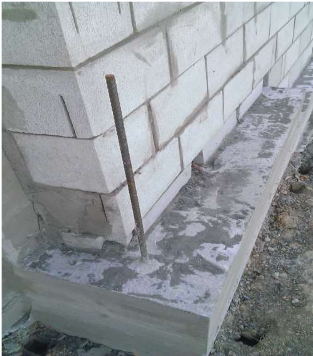
Steel placement incorrect (outside of block wall)
