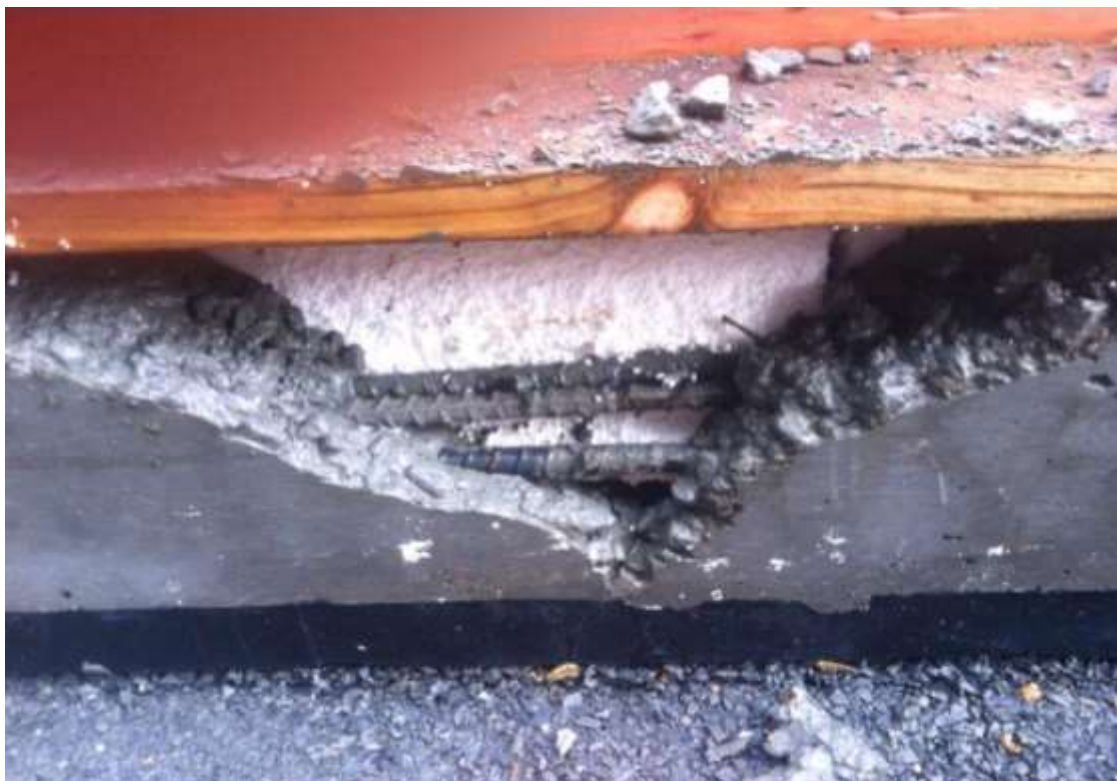
Reinforcing steel exposed at the edge of a slab due to lack of vibration
