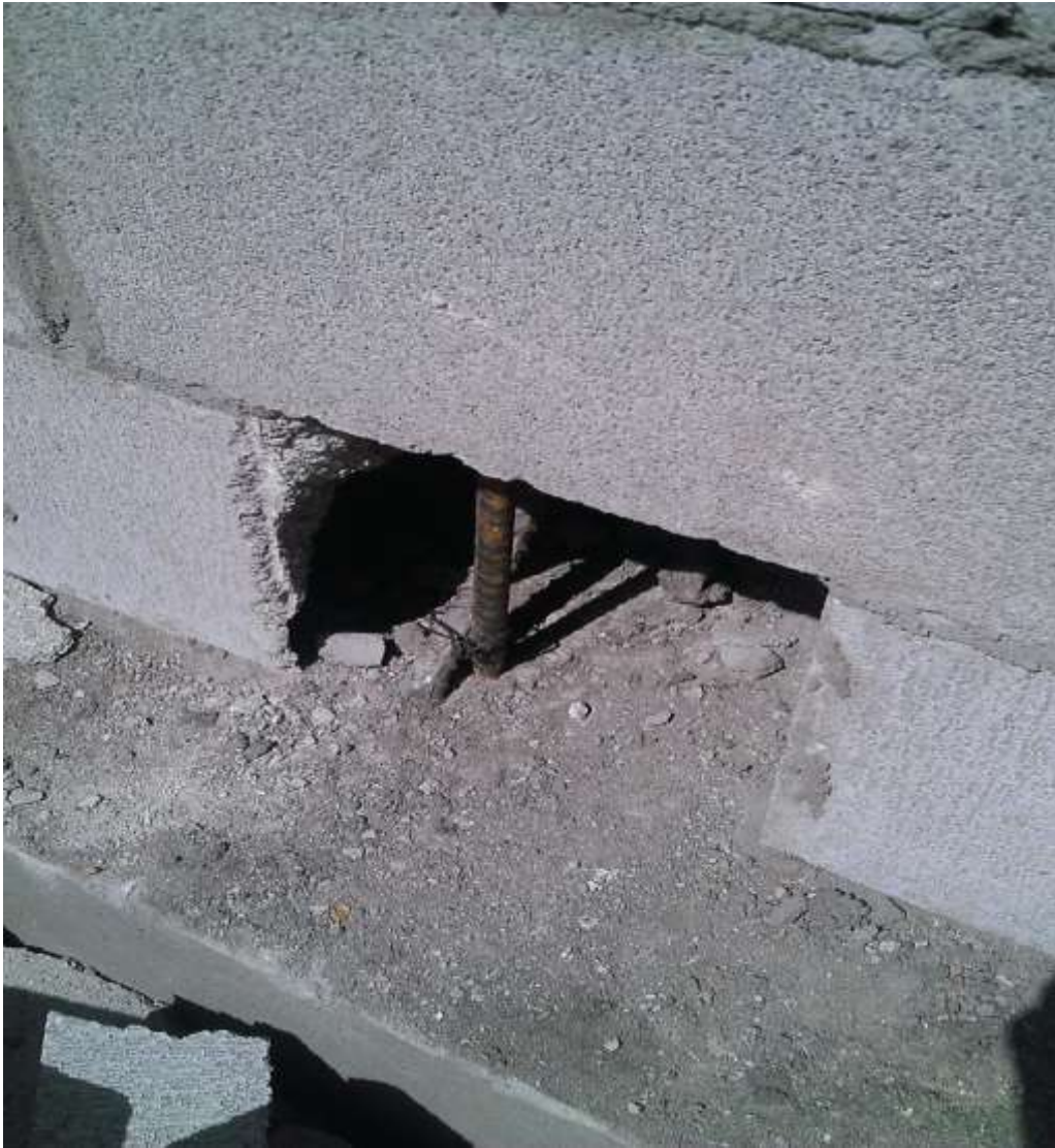
Original steel placement incorrect; steel starter bar bent over and new rod inserted
