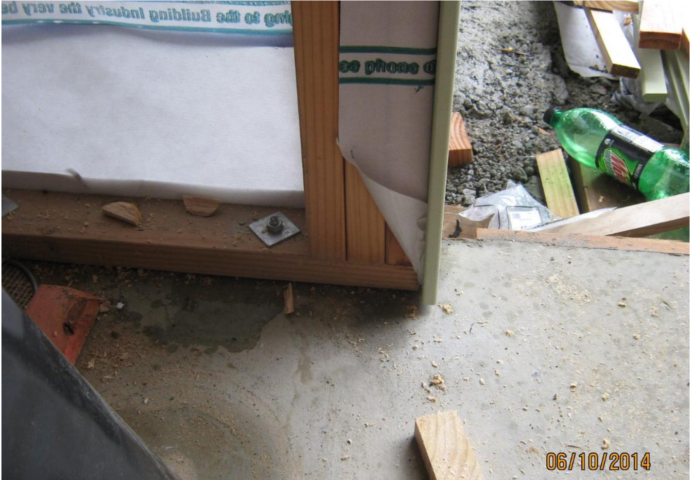
This photo depicts the lintel studs for the above photo; no straps have been fitted at the bottom of the lintel studs. NZS3604 requires straps to be fitted to the bottom of all studs if lintel straps are required. The plan also clearly indicated this.
