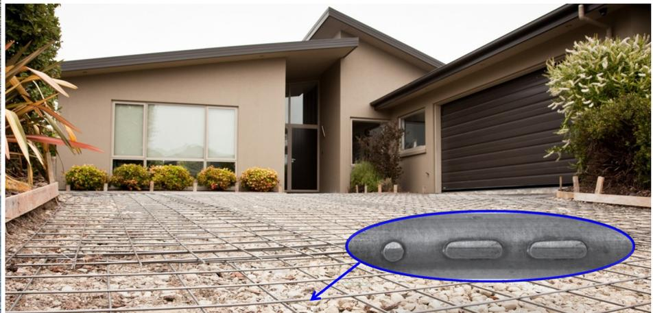
Fletcher Reinforcing uses mesh feed manufactured by Pacific Steel to AS/NZS 4671. Identification of the wire on site is achieved using the wire markings of a single dot and two dashes. The second dash in the 'Dot-Dash-Dash' marking, is a unique identifier of Pacific Steel's SEISMIC® 500E grade mesh feed:
