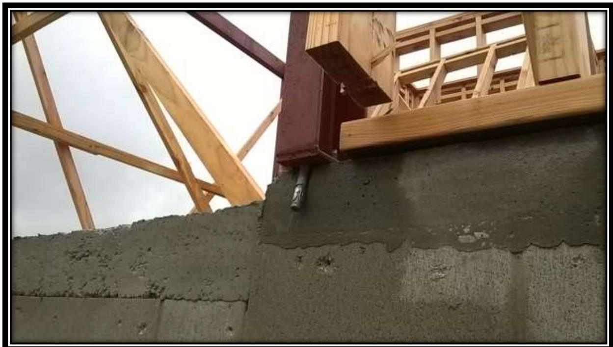
Framing overhanging foundations resulting in inadequate support to framing
